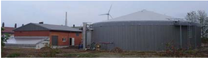
Figure 32: Biogas and wind power plant in Feldheim
