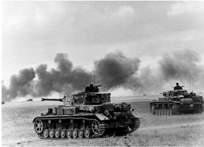
Tanks of the Hungarian Armored Division going into action. These Panzer IV tanks were inferior to the Soviet T-34s, because their maximum hull armor was 30mm. as opposed to 47 and later 60mm. of the T-34s. But their 75mm. guns were capable of knocking them out.
