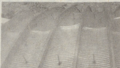
Fig.4. Local buckling of outside test arch
